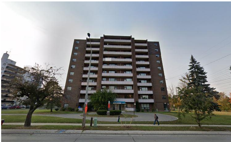
Image of existing conditions facing north
