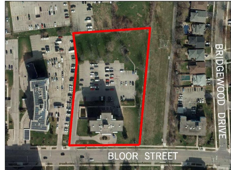
Aerial Photo of 1785 Bloor Street
