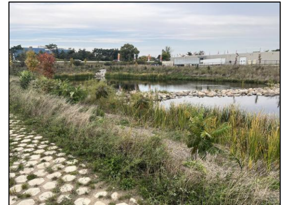
Example 2: Stormwater Management Facility – City of Barrie SWMF SPO3
