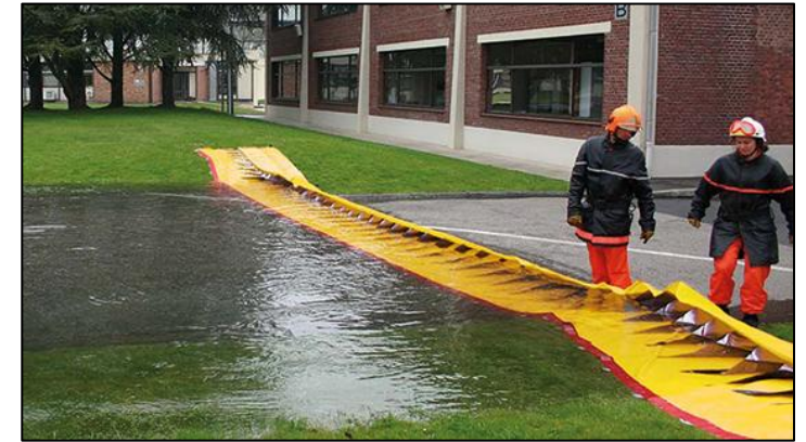
Deployment of Temporary Floodwall
