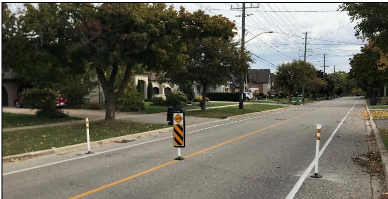
Flexible bollard with flex marker – Glengarry Road
