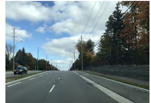
Raised bike lane
